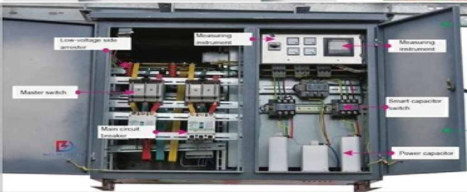
After the installation of the main distribution box is completed, the main internal components need to be checked to ensure that the connections between the internal components are normal, and the installation of the low-voltage integrated distribution box is completed.
